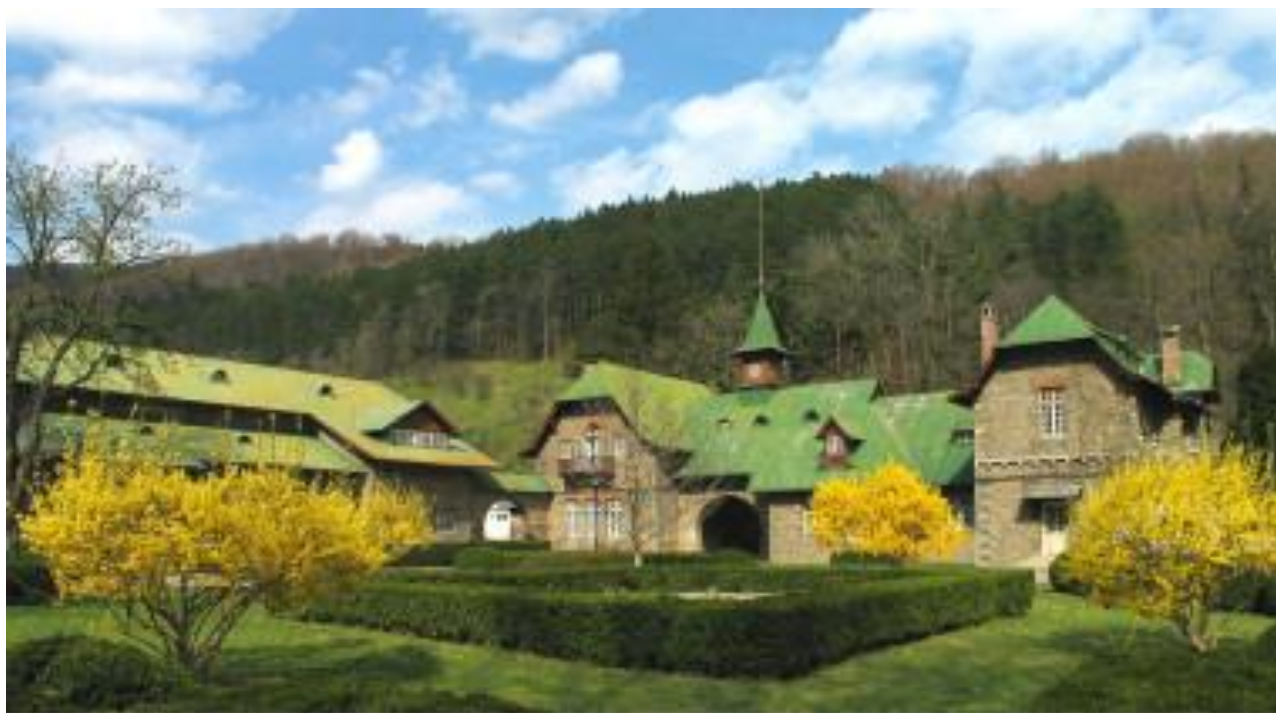
Posada Castle, built between 1842 and 1848 by Gheorghe Bibescu (the reign of Wallachia, known under the name of Bibescu Voda )
